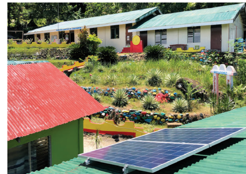
OMF's solar panels installed atop one of the classrooms provide ample electricity to power multimedia equipment, electric fans, and LED lights installed in all classrooms.
